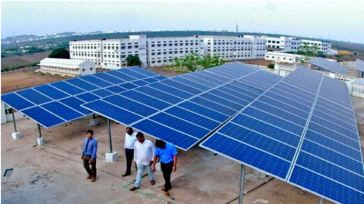
Figure 10 : A Solar roof top system
